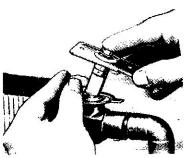
After the valve body has been installed, clean the stem cavity in the valve body, of all foreign matter. It is recommended that a snug fitting round wire brush be used to remove any debris from the cavity.
